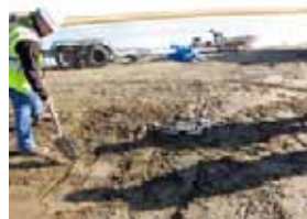
Completed Project – Pile was backfilled with local material
