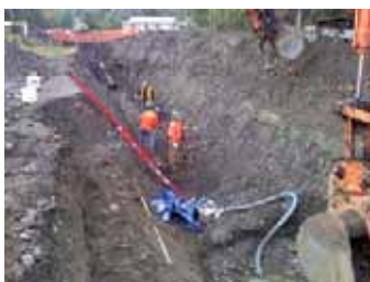
Compacting Pipe Bedding
