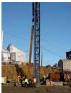
Pile Being Set in Lead
