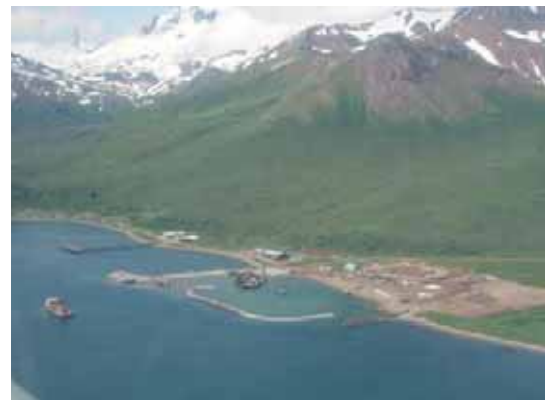
Nearly Completed False Pass Harbor
