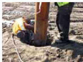
Cutting Pile Below Grade
