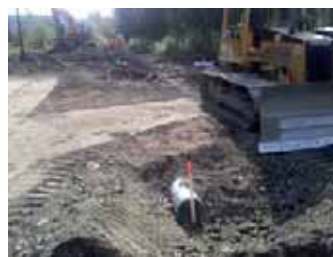
Installing Culverts
